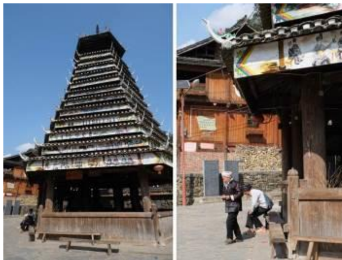
Figure 4. The Drum Tower in Zhanli
