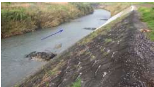
(a) Super dikes of assembled boulders installed in Sakagawa river, Shizuoka Pref.
