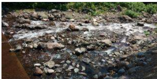
Figure 35. Flow condition at ramp with consecutively assembled boulders in prototype (1/10 slope)
