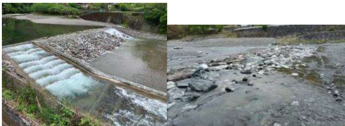
Figure 34. Construction of ramps with assembled boulders and protection region
