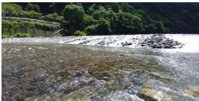
Figure 33. Flow condition at ramp with consecutively assembled boulders in prototype (1/4 slope)
