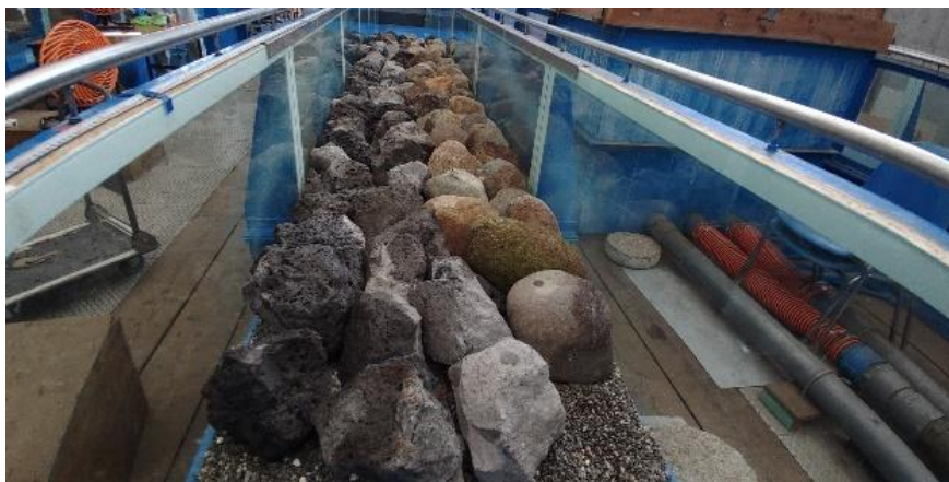
Photo 2. Installation of assembled boulders (left side Slag)
